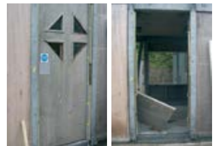
Fire Door - Before & after
